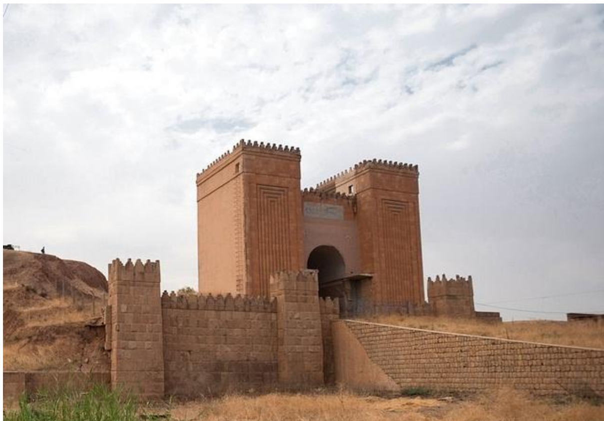
The Mashki Gate at Nineveh
